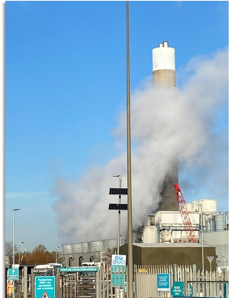
Current Energy from Waste facility emitting heat (steam) to atmosphere
