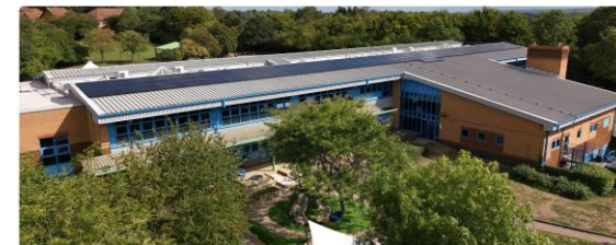
Solar Panel Installation at West Grove Primary School
